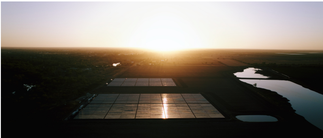
Latitude (foreground) and Chillamurra Solar Farms, Boggabilla NSW
